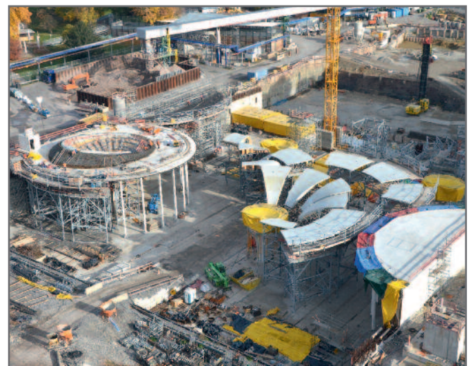
Construction project S21: Support for the concrete goblet shape towers
