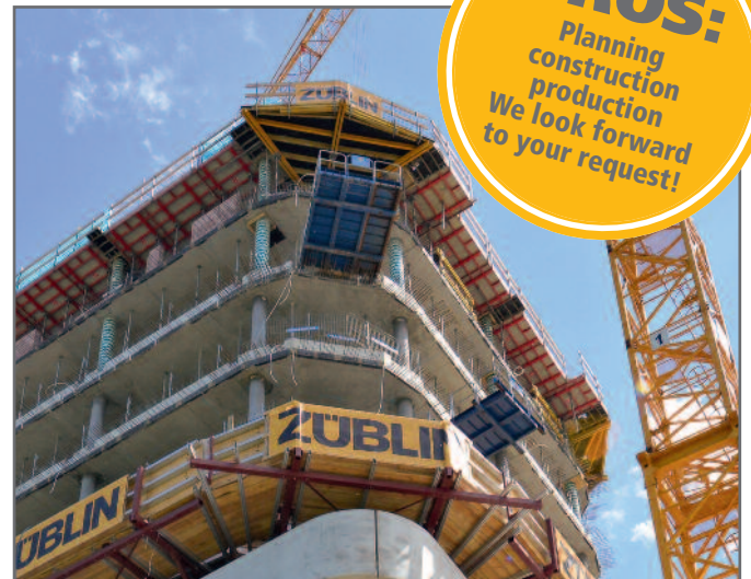
BV SKY Bietigheim: Special working platforms
