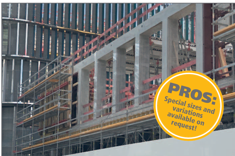
Steel frame, all sides formed conical
