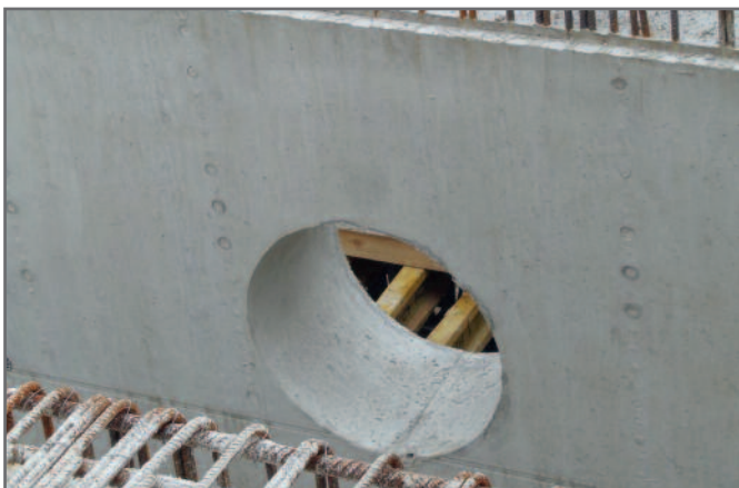
Easy use when concreting girders: the flex-forming tube can be drawn out after loosening the wedge segment.
