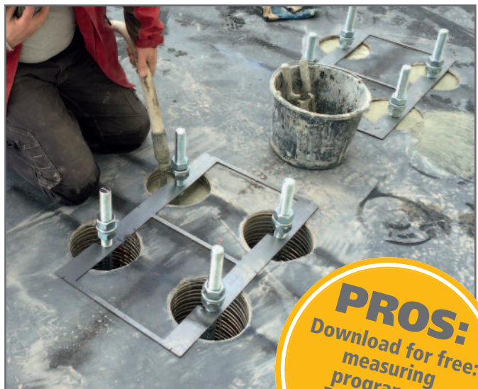
Grouting the anchor bars
