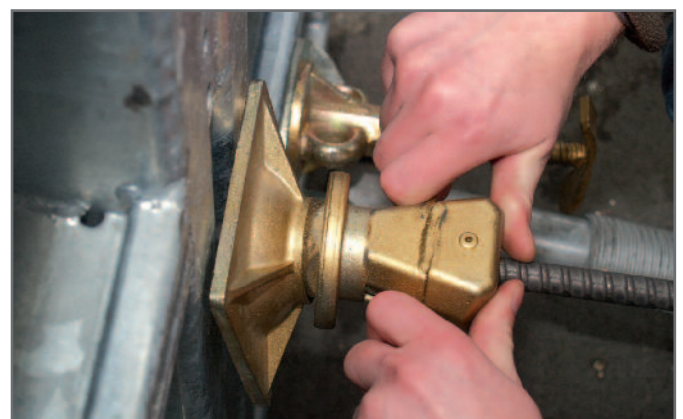
Thereafter, the Rapid Locking Nut can be pushed over the bar, holding the wings simultaneously.
