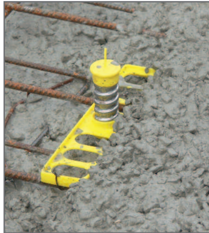
Before concreting: with installation kit D&W 20 mm
